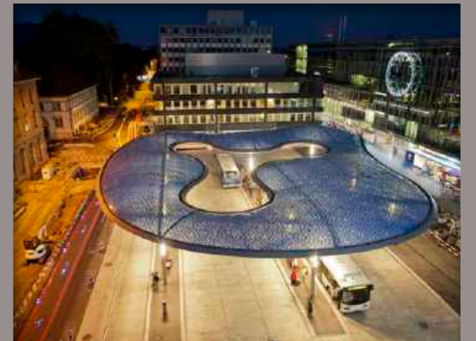
4. Aarau Bus Station canopy
